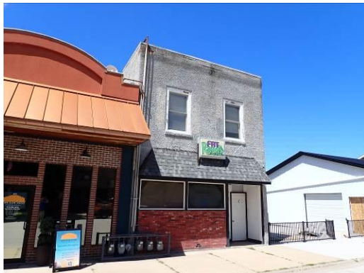
1. View from the southwest
