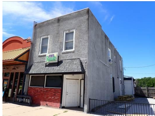
2. View from the southeast
