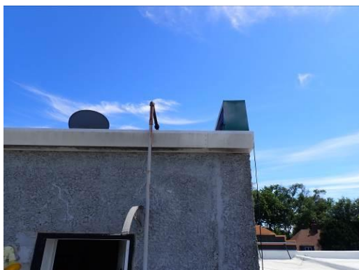
35, 36. Views of gutter on north side
